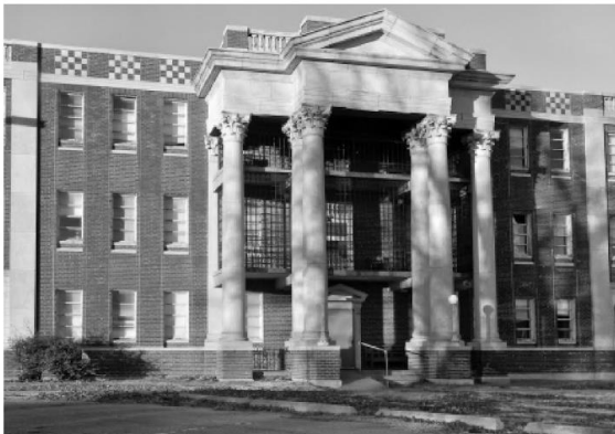
One of Hope Hall's entrances. Wheelchairs rest on the caged balcony.
